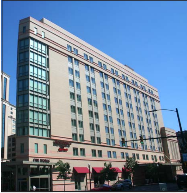
The Residence Inn Arlington Courthouse is a limited-service hotel
