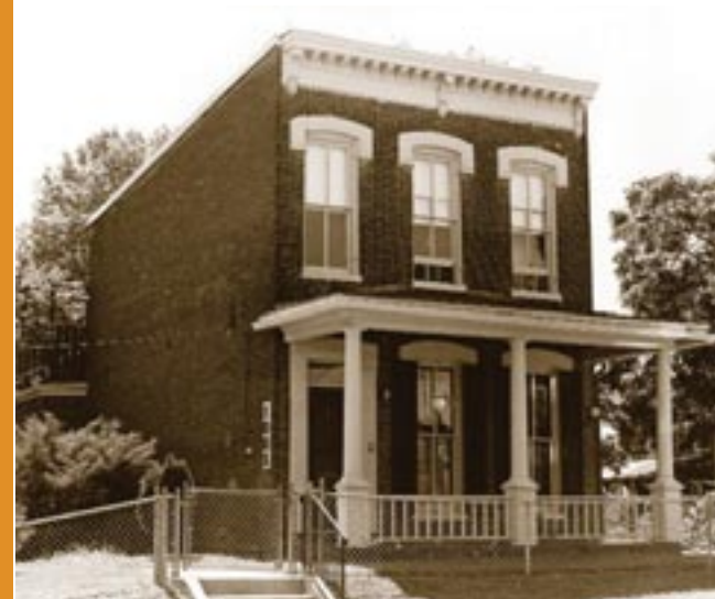
Harry W. Gray modeled his home after townhouses he had seen in Washington's Foggy Bottom neighborhood. Learning masonry as a slave at Arlington House, Harry applied his skill to building the first red brick townhouse in Arlington County in 1881. Photo provided by Arlington Historic Affairs Landmark Review Board.
