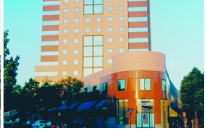
This building in the heart of Clarendon is illustrative of conflicts between security and the urban village concept
